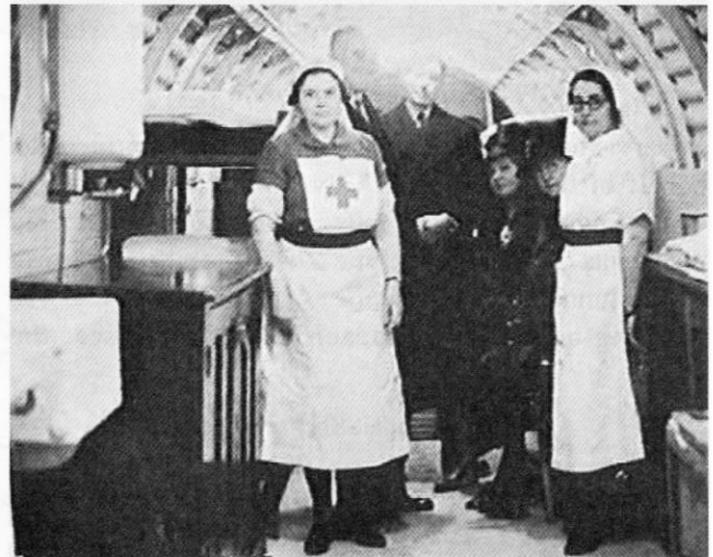
First Aid Post in Wymering Shelter
